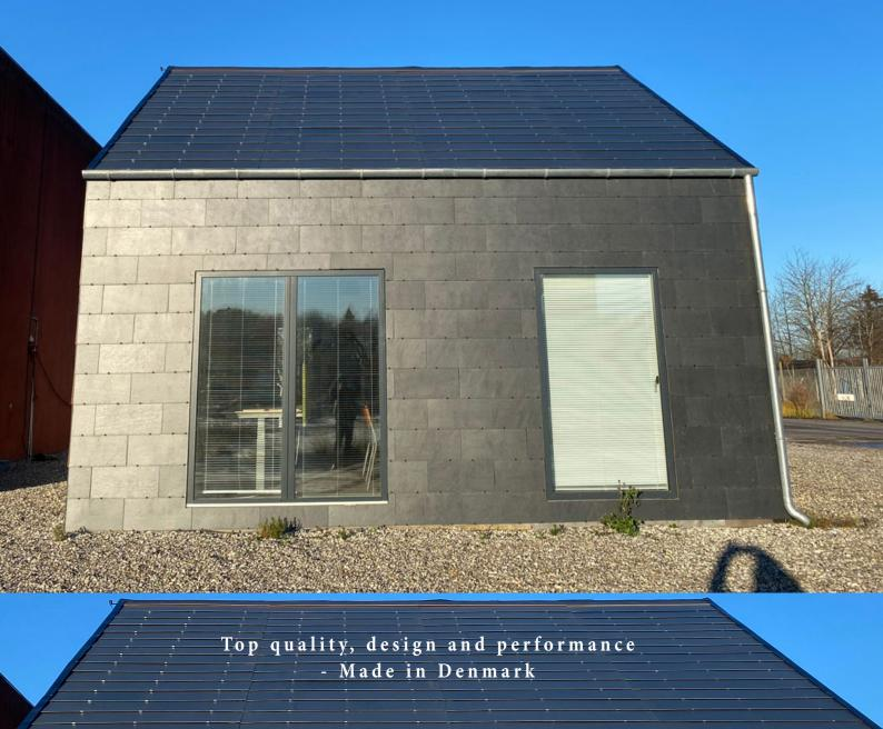
A solar roof - project in Hedehusene at Rockwool's headquarters in Denmark, combining solar PV and insulation.
