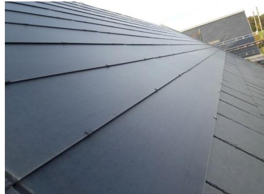
Is a unique new patented building integrated (BIPV) mounting system, which also makes it possible to integrate Danish Solar Energy CFR modules into roof surfaces such as slate roofs, where you do not have to do a whole new interior construction to preserve roof aesthetics. The low height of this solution allows you to settle for only the areas on which the CFR modules are intended to be mounted. Mounting can be supplied so that it does not fill more than 6 mm in height.
